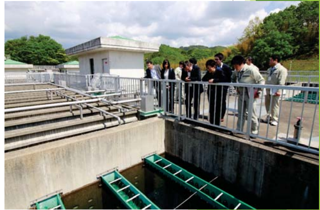
Arai Water Purification Plant Water and Sewerage Bureau
