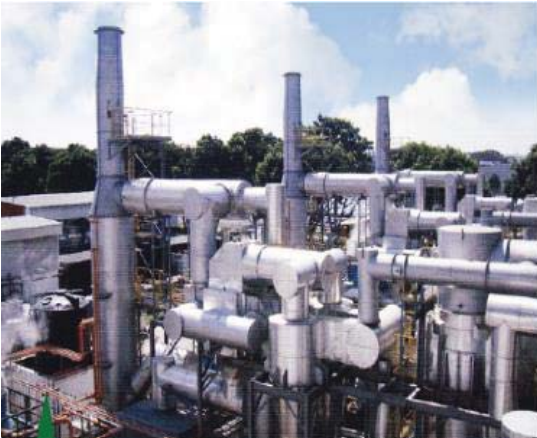
Plant in Singapore Largest Sludge Processing Plant Equipment in Southeast Asia
