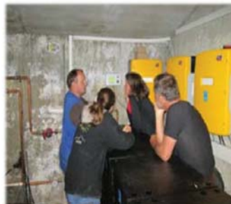
Manager of the Hutte and installer
