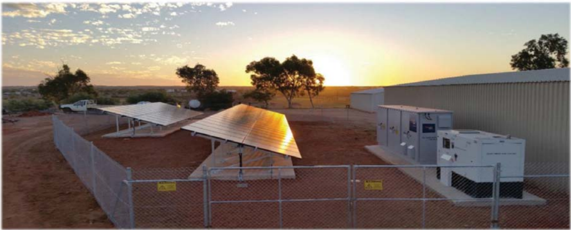
Effective use of solar power and electric generator power
