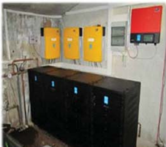
Batteries and SMA Sunny Island
