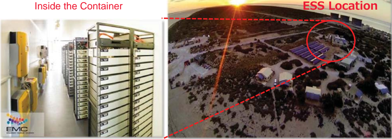
330 kW solar PV, 620 kWh lithium energy storage, 4x100 kVA diesel
